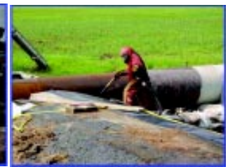
Fig 15 – Grit blasting in operation.
