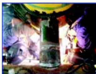
Fig 23 – Reinstating the support clamp over the composite repair.
