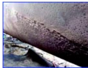
Fig 14 – Manual excavation and surface preparation.
