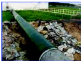
Fig 20 – Application of final corrosion coating.
