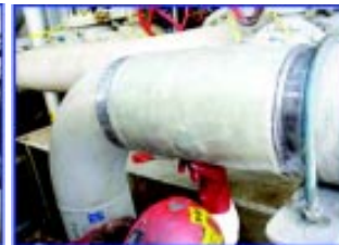
Fig 10 – Inspection of each repair layer as applied.
