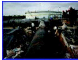
Fig 14 – Manual excavation and surface preparation.
