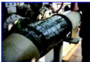
Fig 11 – Application of peel ply.
