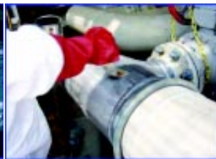
Fig 8 – Wetting of pipe surface.
