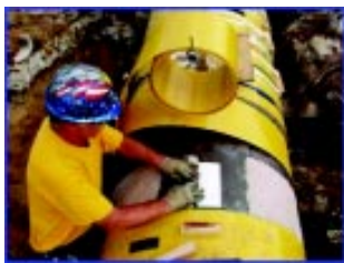
Fig 17 – Application of filler into defect.
