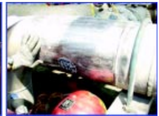
Fig 6 – Leak sealed and completed surface preparation.
