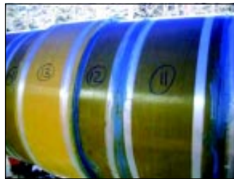
Fig 4 - Girth Weld, bridging technique repair
