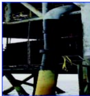
Fig 23 – Reinstating the support clamp over the composite repair.
