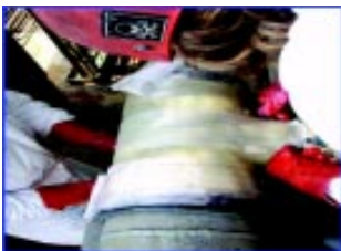
Fig 11 – Application of peel ply.
